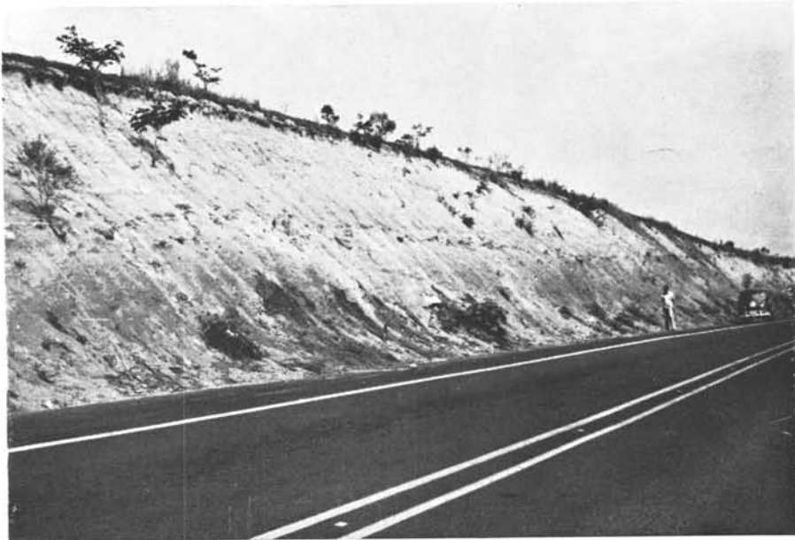
Fig. 3. General view of upper boulder pavement on southern face of road cut.
