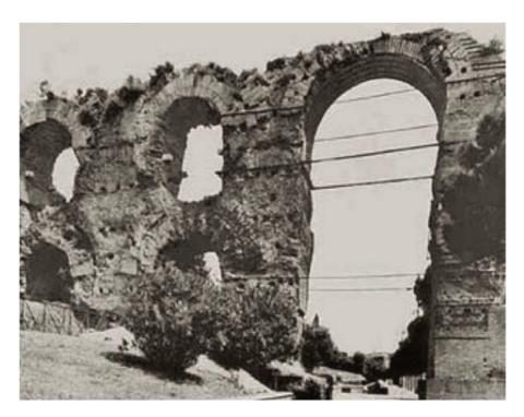
Figure 2 The Aqua Claudia, built between 38 and 52 AD, measuring 69 kilometers in length and channeling a volume of 184,220 m<sup>3</sup>/day (2,132 L/s)
