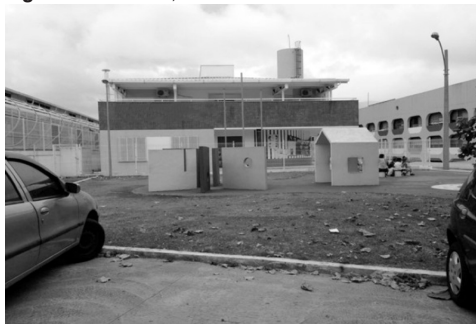
Figure 9- School 4, front view.
