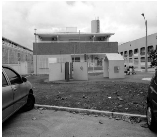
Figure 51- Front view of school 4.
