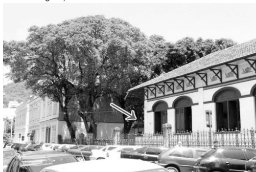
Figure 28- Front view of School 3 - opened in 1909 - (arrow indicates gate).
