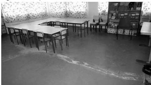
Figure 26- Repair in cracks on the floor of School 7.
