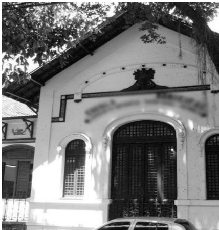
Figure 50- Front view of school 3.
