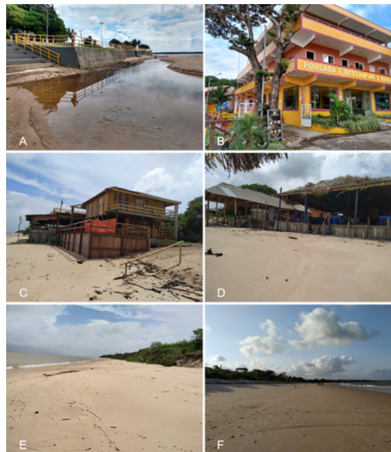
Figure 3. Artificial structures (A, B, C, and D) in the northwestern sector and natural protective structures in the southeastern sector (E and F) on Praia Grande beach. Photographs taken 05/02/2021 (A and B) and 9/13/2019 (C-F)
