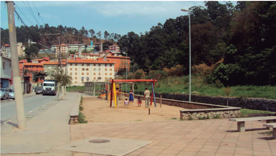
Image 7 - Hugo Ítalo Merigo Street after the opening of linear park: asphalted street, wide sidewalks, equipment of leisure, enjoyment and channeled stream by gabions. Photo by Wellington Tohoru Nagano, 2014.
