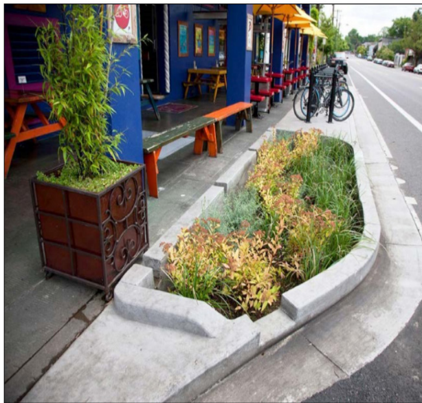
Figure 7 – Green gutters are landscape areas on the side of the street that store, filter and infiltrate the runoff of rainwater.
