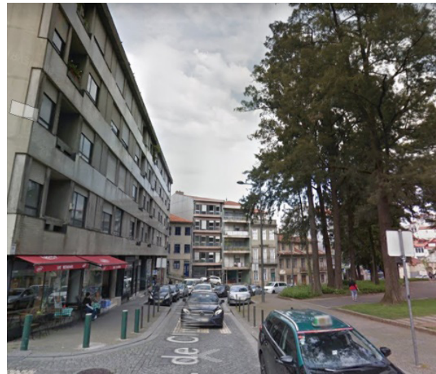
Figure 6 – Physical survey of the item “soft borders”.
