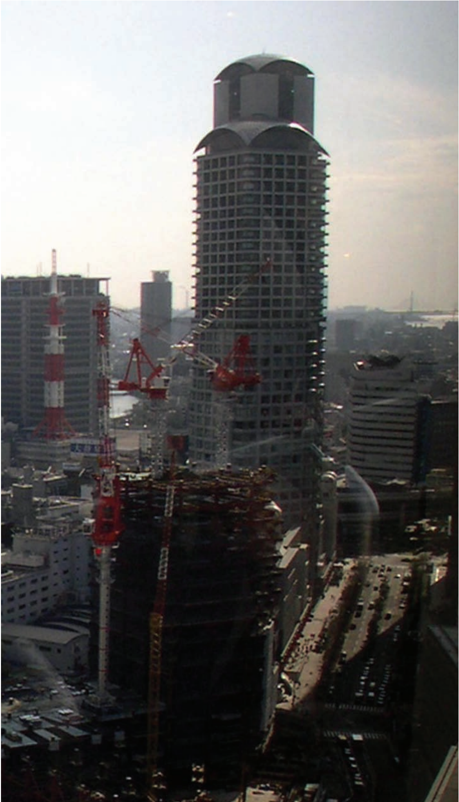
Photo 3.2: The tower of Herbis Osaka and sidewalk widening
