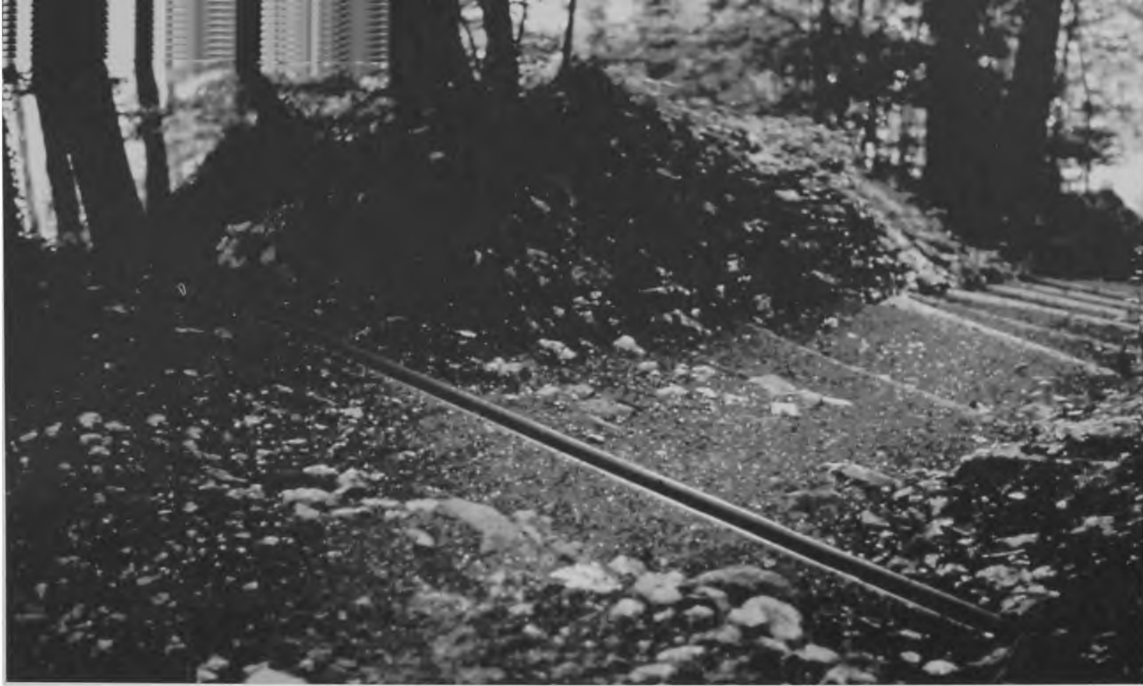
Figure 17. Voie Suisse, Lake Brunnen, Switzerland, 1990. Georges Descombes. The earthen path reinforced by stainless steel drainage channels. [Marc Treib]
