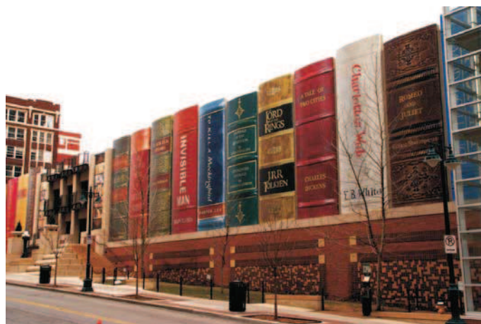
Figure 3: Library Parking Garage. Source: Crest (2014).
