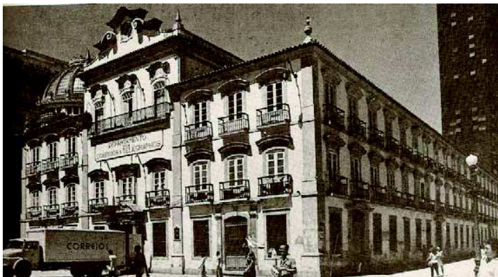
Figure 16: Paço Imperial before intervention. Source: CAMPOLLO, 1984, p.141.
