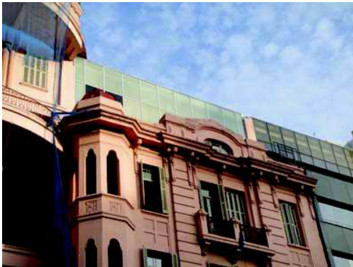
Figure 7: Mário Quintana Culture House: posterior facade where the cover was incorporated in metallic structure and glass. Source: Photo by the author.
