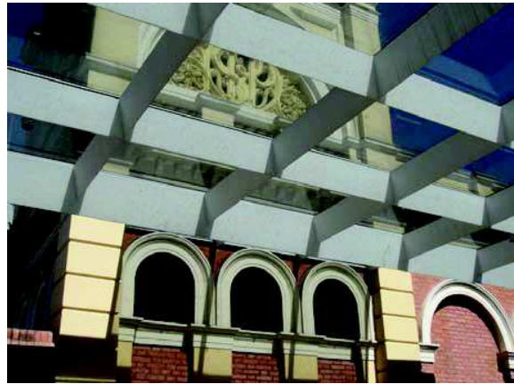
Figure 21: New metal cover of Museu da Língua Portuguesa, at the entrance of Luz Station. Source: Photo by the author.
