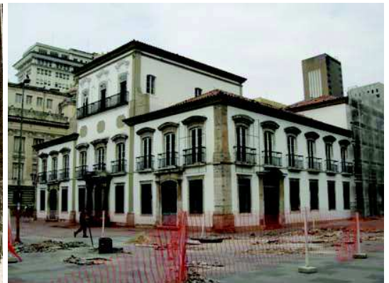
Figure 17: Paço Imperial Culture Center after intervention. Source: Photo by the author.
