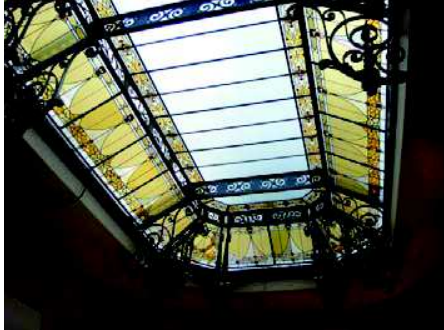
Figure 13: Positioning of the Dome on the last floor of the Banco do Brasil Culture Center. Source: Photo by the author.
