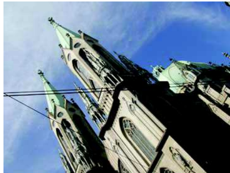
Figure 24: Sé Cathedral highlighting the new turrets and needles executed according to the original design. Source: Photo by the author.
