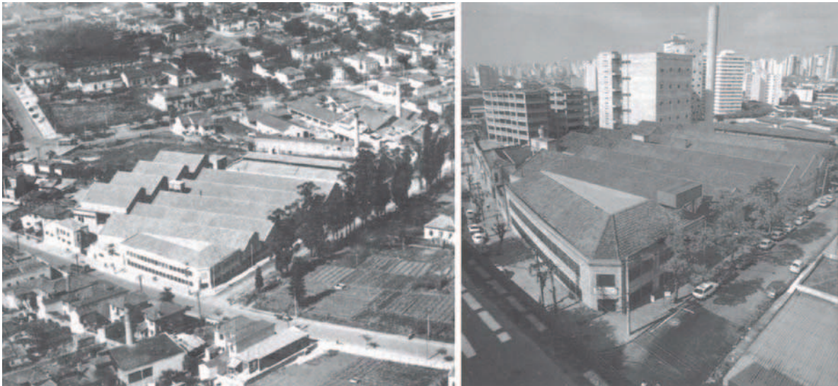
Figures 4, 5: Aerial views of assembly: before and after the intervention
