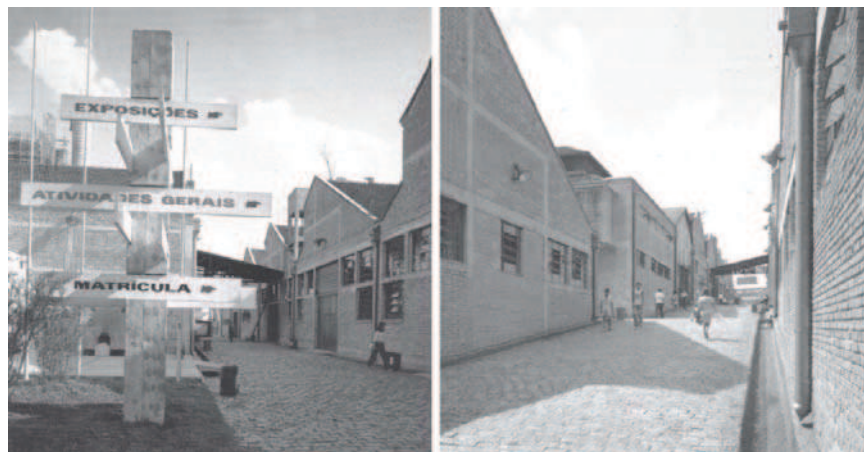
Pictures 6, 7: Totem and inner street with rolled pebble channels. Source: VAINER and FERRAZ, 1996, p. 66 / FERRAZ, 1993, p.223.
