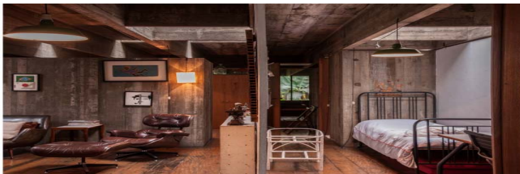
Figure 10: View of the living room and bedrooms, in which the distance between the closures and the slab can be observed. Source: Photo by Lauro Rocha.
