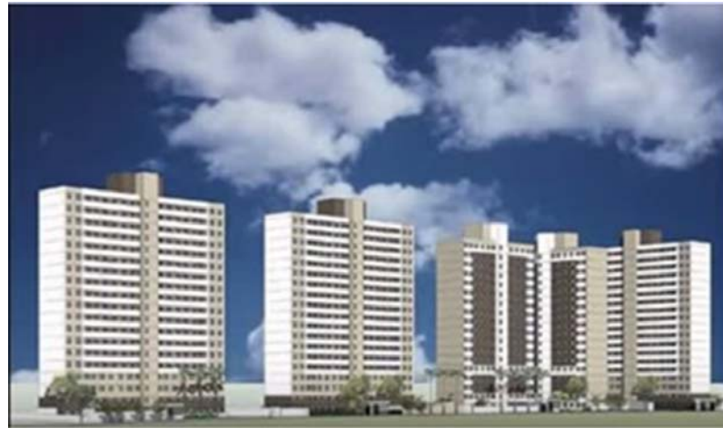
Figure 4: HIS and HMP in ZEIS 3 Barra Funda – “BARRA VIVA” development 5 towers and 953 UH. Source: flyer.
