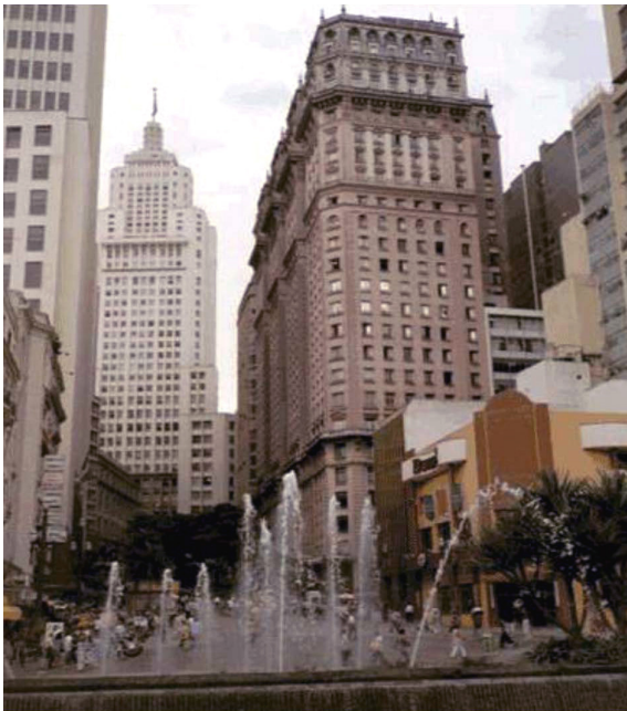
Figure 2 - Martinelli Building Source: https://www.prediomartinelli.com.br/fotos/fotos.htm
