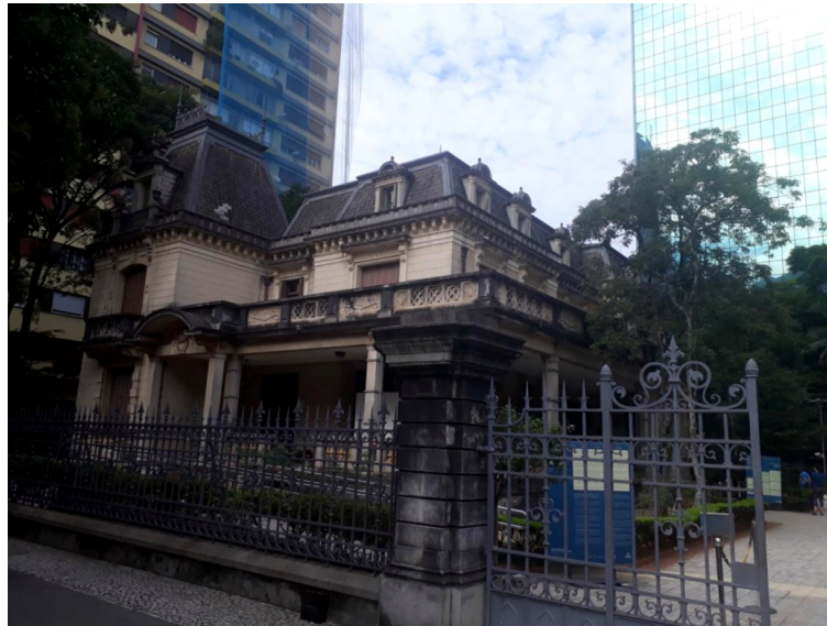
Figura 2: Casa das Rosas and Parque Cultural Paulista Building (the glass tower) Source: the author, 2019.
