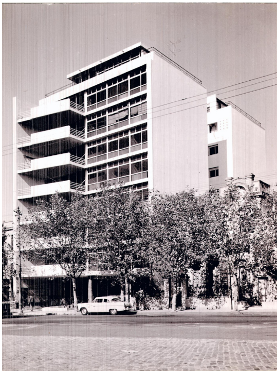
Figure 2 – García Pardo. Photo of the Gilpe building Source: García Pardo Archive – Institute of History, Facultad de Arquitectura, Diseño y Urbanismo [192-]. Photograph b&w
