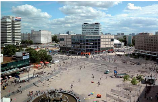
Figure 9: Electronics Store in front of “Haus des Lehrers”, destruction of the sight-axis. Source: Philipp Eder.
