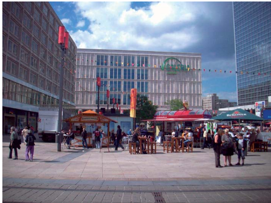
Figure 10: “Alexanderplatz”, replicated facade at “Kaufhof”. In front: razzle dazzle instead of a public space. Source: Martin Gegner 2010
