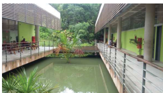
Figure 4 – Inside view of Educational Center Burle Marx Building. Source: Author's photo
