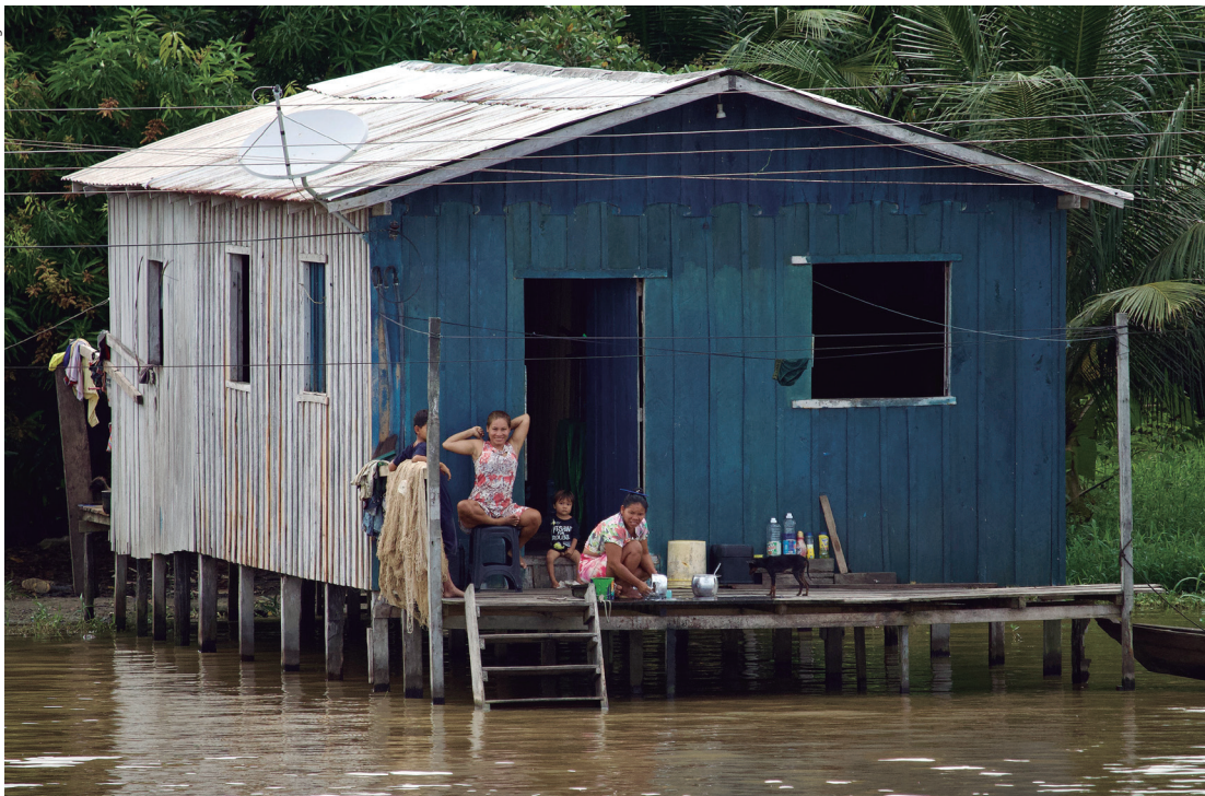
Uma típica casa de ribeirinhos no Rio Solimões. A estrutura de palafitas protege as casas durante a cheia dos rios A typical riverside home in the Solimões River. The still structure protects the home during the high-water season
