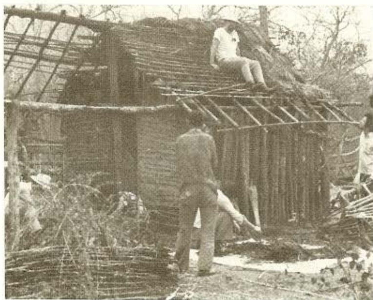
Fig. 1 — Residence FLG I A . Note to the right of standing man the open wall of wooden stakes not favourable for bug colonization and the mud cowdung wall to the left of him suitable for bug colonization
