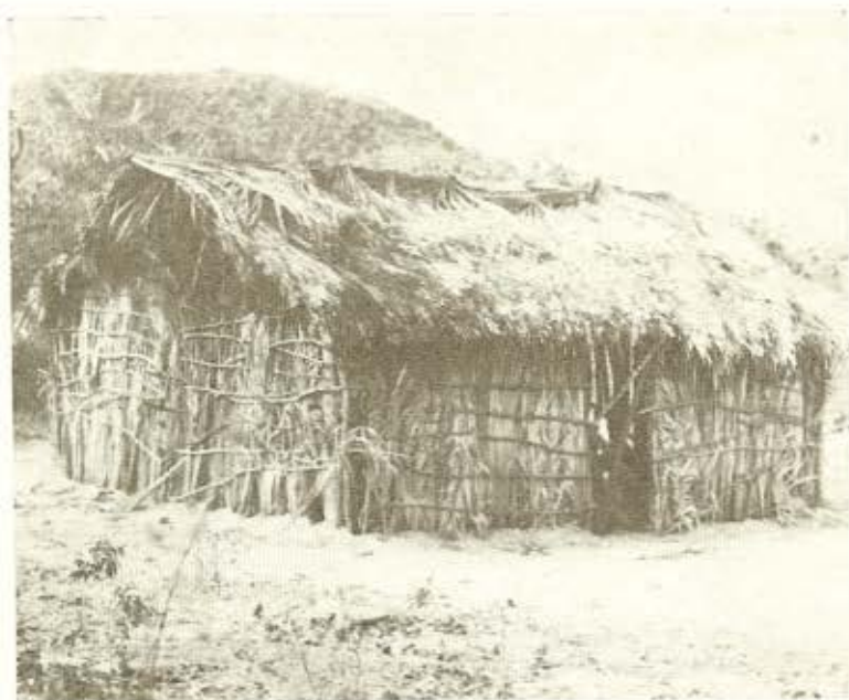
Fig. 3 — Residence UnB 2 constructed entirely of palm. Note the fan shaped buriti palm fronds forming the roof crown
