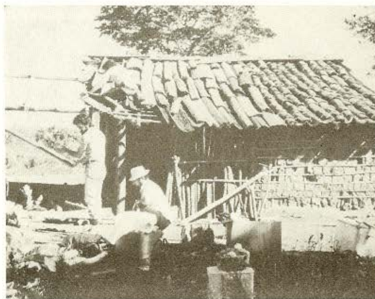
Fig. 2 — Residence LN 3. Note roof composed of two different tiles. To the left the bark of the imbirusu tree and to the right portuguese ceramic tiles
