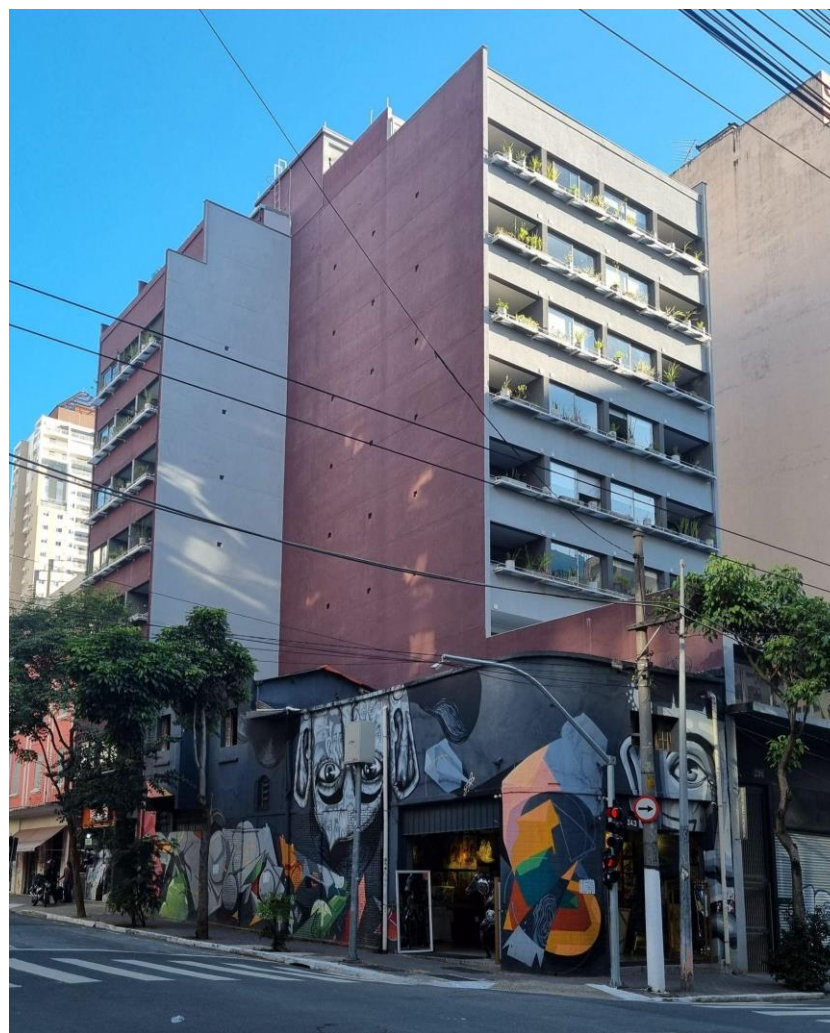
Fig. 7: Corner of Marquês de Itu Street and Rego Freitas Street, São Paulo, Brazil. Source: Mariana Lunardi Vetrone, 2024.
